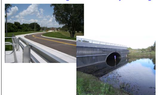
As part of the City of Lakeland's Recreational Master Plan, JSK worked together with the City and the Lakeland Regional Cancer Center to design, engineer and permit the construction of this jointly funded project. The project involved installing a culvert crossing over Lake Crago Canal as well as the construction of over 1,200 linear feet of 8-inch and 12-inch water main to help extend the City's existing potable water distribution system.
